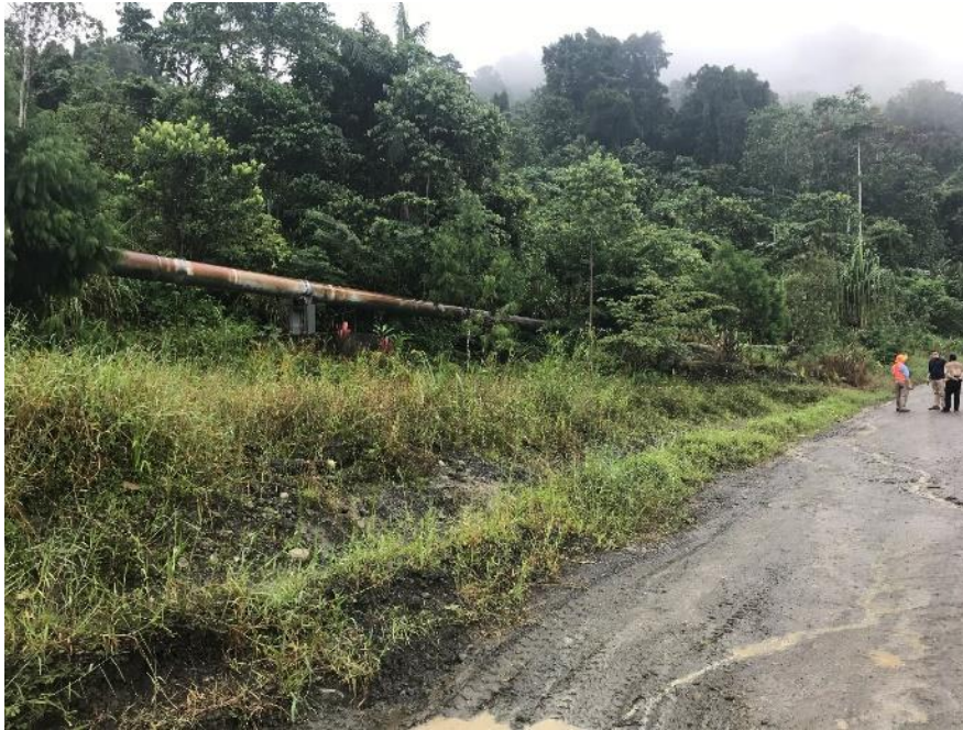
Figure 5-7 Ramu Nickle Slurry Pipeline
